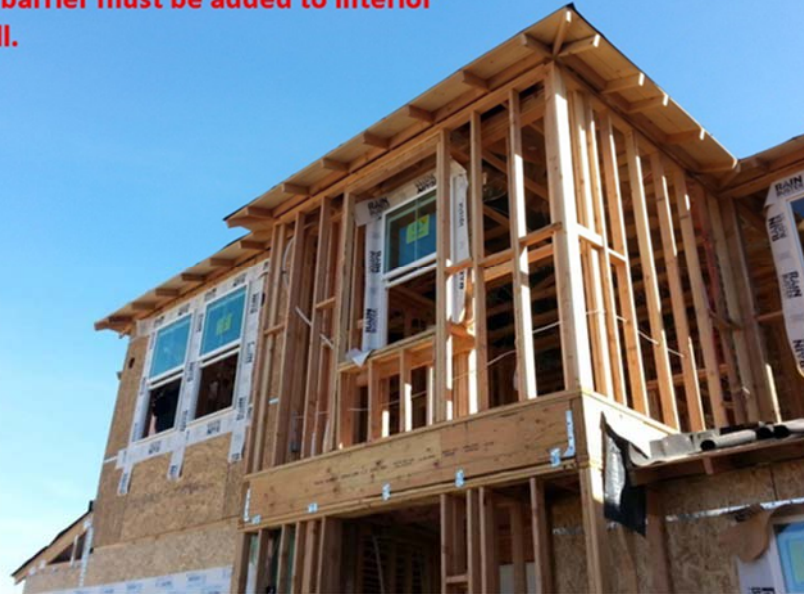
Figure 2 In this example it would be best to insulate the interior wall. An air barrier must be added to the interior wall that is sealed to the bottom plate, top plate, and all penetrations sealed. Ensure interior bottom plate is sealed to subfloor.
