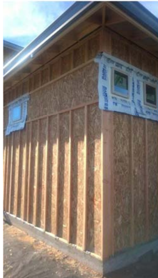
Figure 1 In this example 2 inch spacers are added to the exterior air barrier. Insulation is only required on the interior side of the air barrier not between the spacers.
